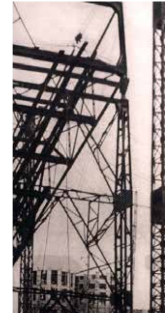
Maks Al'pert, Coke chemical plant. A sloping shaft for coal feeding. Photo © Maks Al'pert
